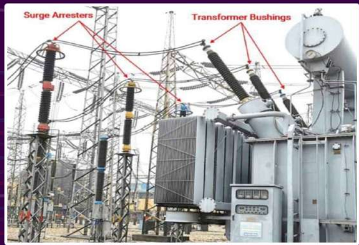
Surge arrester working principle
